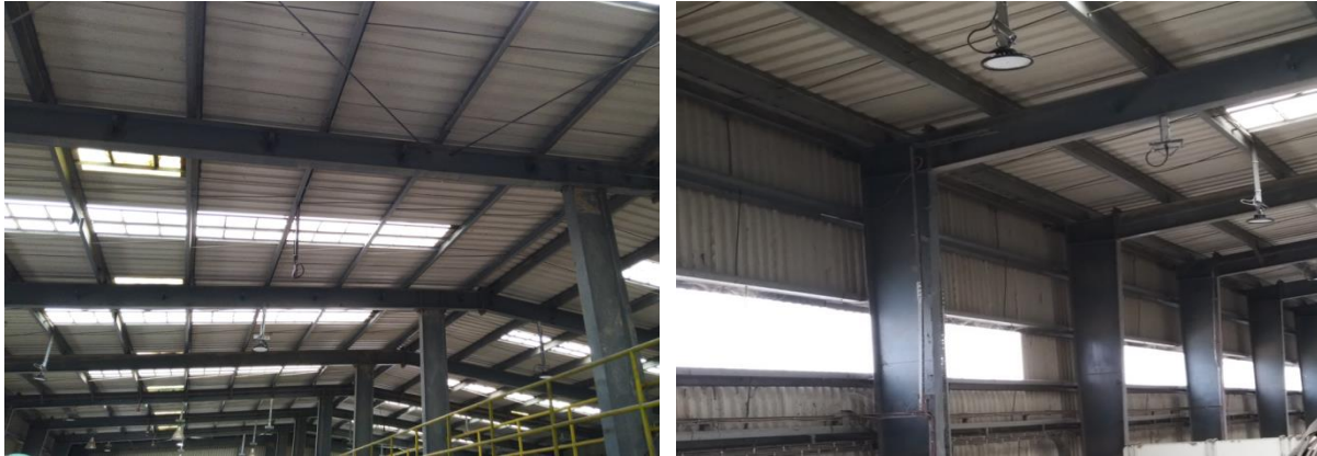
Figure 4: Pitched roof support structure
